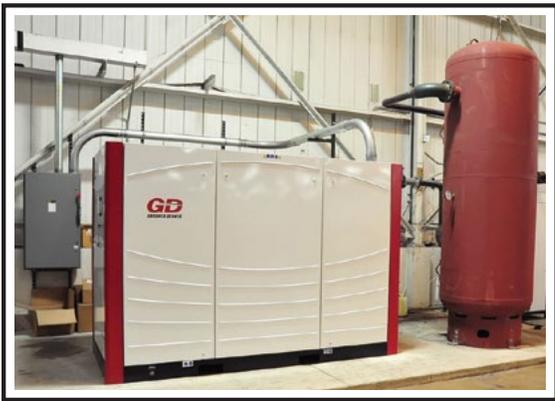
But when Tribune Direct analyzed the option, projections showed that running two 150-HP compressors would cost around \$130,000 for the nearly two million kilowatt-hours (kWh) used per year. While this was a good solution, Craig Sipich, director of technology and engineering at Tribune Direct, wanted a more energy-efficient solution.
